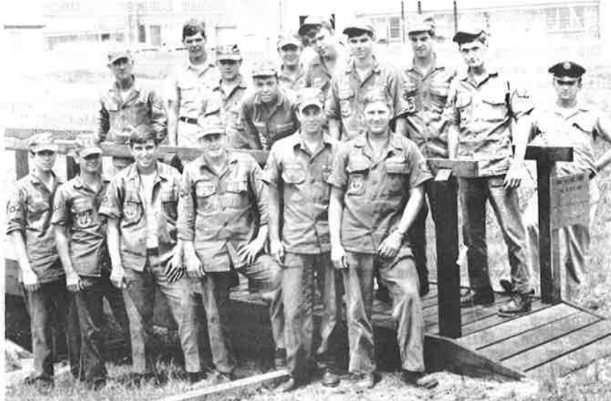
Shown above are members of the 192d Tactical Fighter Group Civil Engineers standing on "The Bridge Over the River Dry". This massive structure was built within 24 hours during Annual Field Training at Travis Field, Savannah, Georgia. Lt. D. F. Caskie designed the bridge and construction supervision was conducted by TSgt Cecchini. The bridge which is 28 feet long, was constructed behind the Dispensary at Travis Field. A sign was placed at the foot of the bridge stating--"The Bridge Over the River Dry built by Valdrighi's Raiders, July 1969, VaANG."
