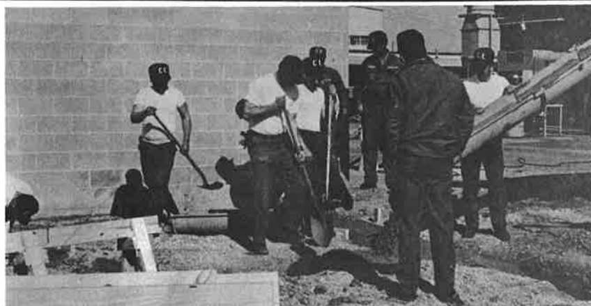
192d CE guardsmen pour concrete for footings of a four bay wash rack the unit constructed as one of four major projects completed at Dannelly Field, Alabama, during the unit's annual field training.
