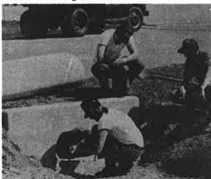
Workers check out storm sewer
