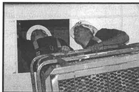
Master Sgt Don Matney and Senior Airman Ryan San Nicolas are pulling wire through the suspended ceiling in the hangar to support the new surveillance camera system the Communications Flight is installing on base. The new system will cover key locations on base with 24 hour video surveillance.
