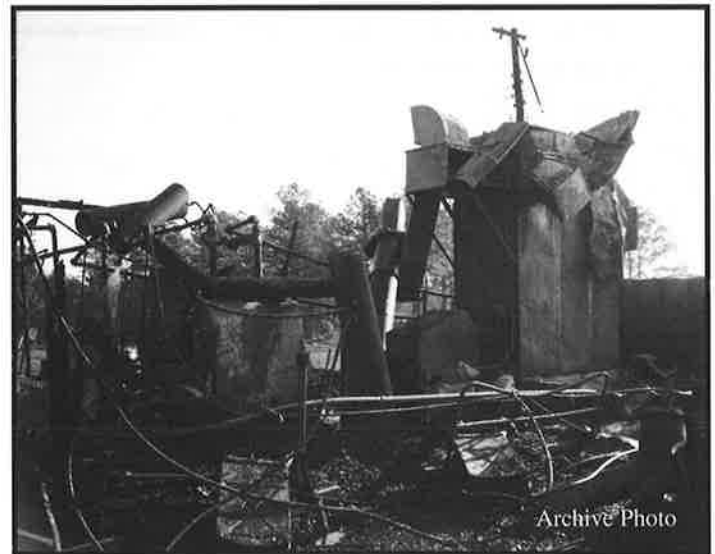
These are the remains of a boiler damaged in the fire.
