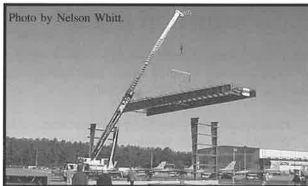
CE folks Lifting 1 st steel beams and purlins into place for the new alert shelters.
